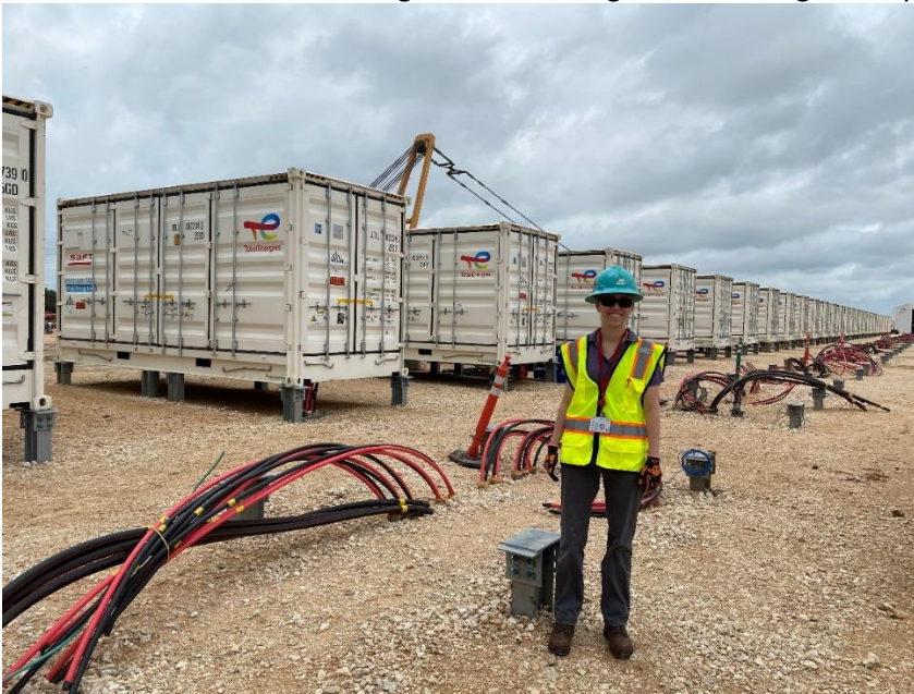
Batteries being installed at a 225 MWh BESS project site in Texas
